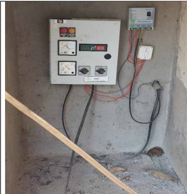
Level sensor of pump with starter
